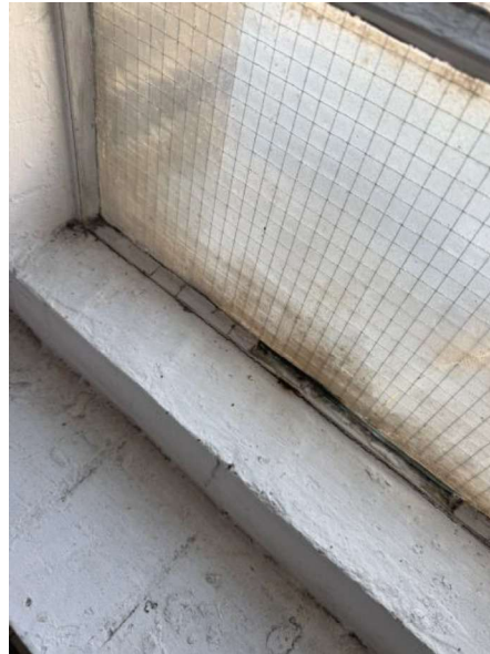
Cracked glazing putty at the sill.
