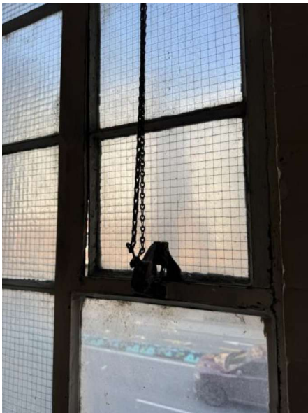
Operable awning sash not fully seated in the frame due to worn or ineffective latching hardware.
