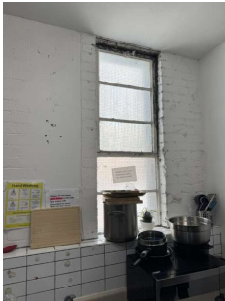
Atmospheric soiling and partially missing hardware mechanisms.
