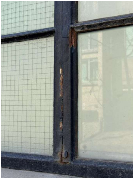
Minor corrosion at exterior of the mullion.
