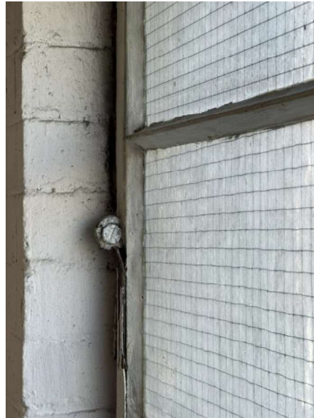
Stress cracking within interior frame members.
