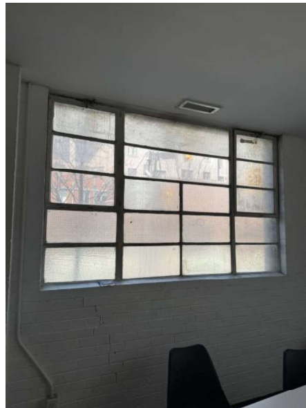
Replaced and original glazing.
