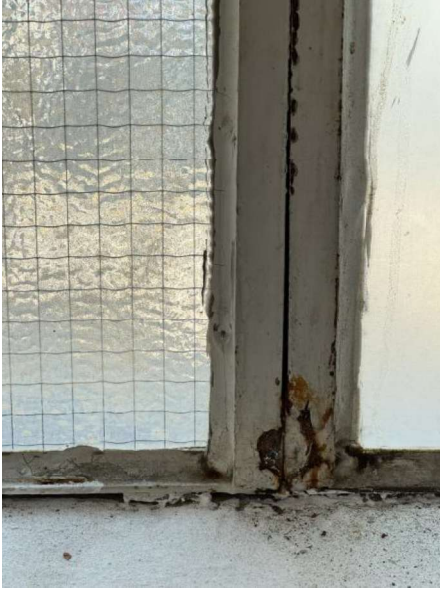
Minor corrosion at sill and cracked glazing putty.
