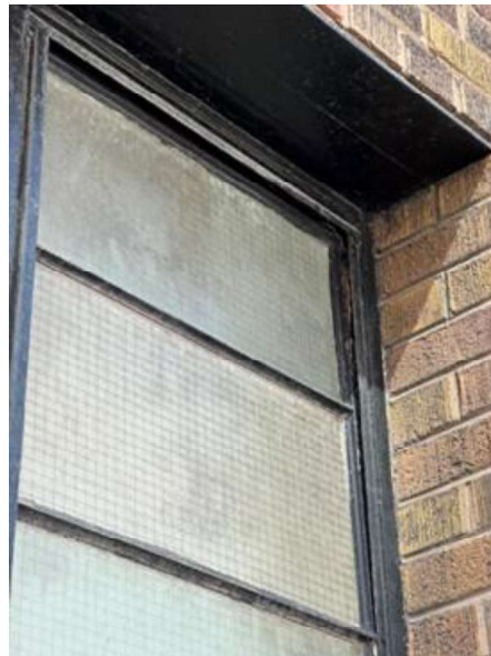
Minor corrosion at operable sash.
