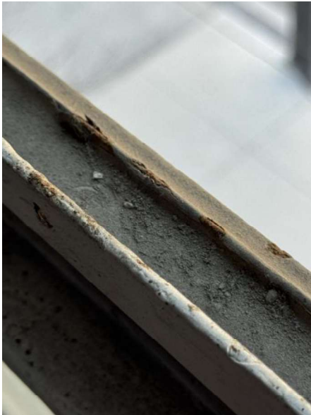
Minor corrosion at the bottom mullion of operable sash.
