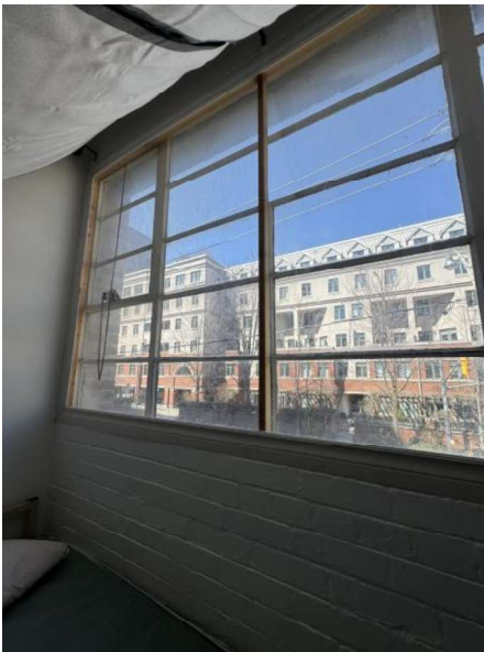
Window with interior storm and complete glazing replacement (Bedroom 204).
