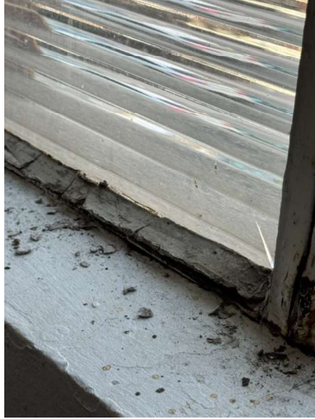
Cracked glazing putty and minor corrosion at sill.
