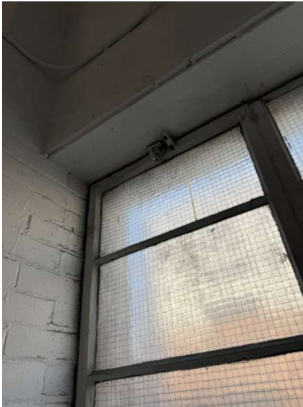
Partially missing hardware mechanisms.
