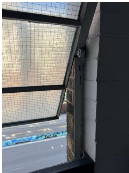
Double height window horizontal pivot hinges.
